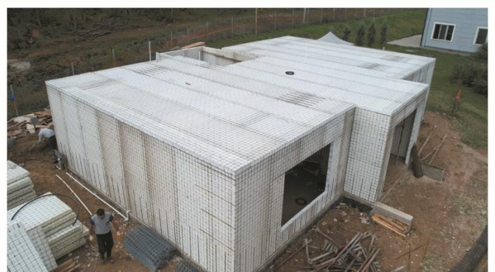
Zenon Panel system performs a monolithic structure behaviour Performs excellent earthquake resistance.
