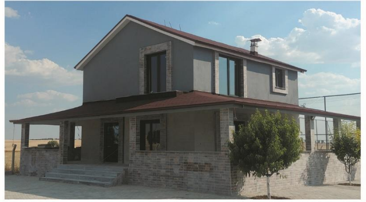
Zenon Panel Structures' static behaviour is monolithic, all walls transfer the load linearly to the ground.
