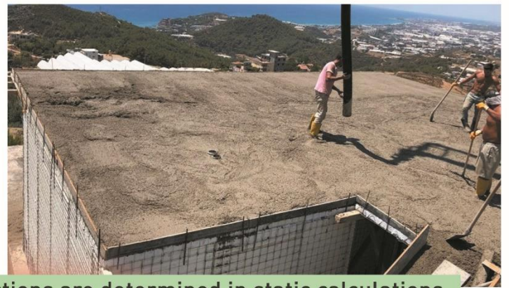
Steel rebar is tied and concrete is poured. Sections are determined in static calculations.
