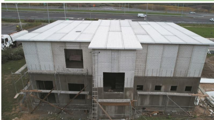
Zenon Panel system performs a monolithic structure behaviour Performs excellent earthquake resistance.
