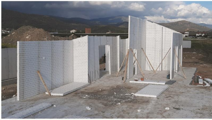
Panels are cut according to the project dimensions. All panels are connected to each other with meshes.
