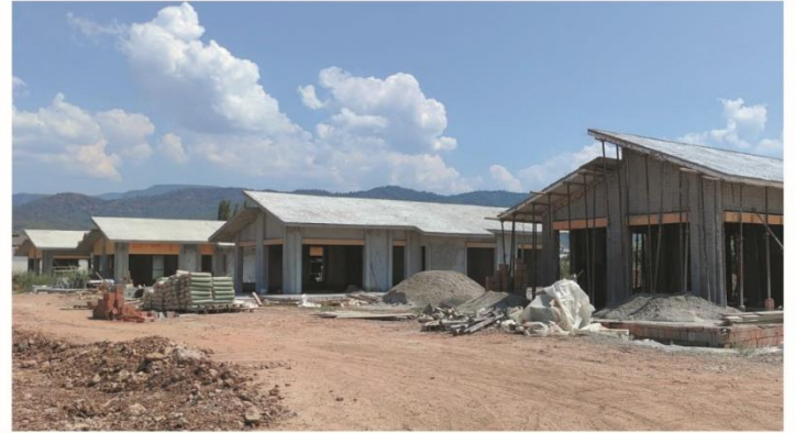
Both wall faces are being shotcreted with cement based mortar. Concrete is poured on the slab.
