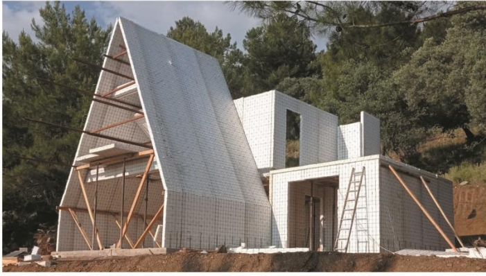
After the concrete is poured, any kind of waterproofing material can be applied.
