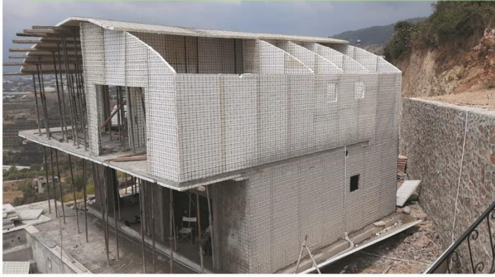
Steel rebar is tied and concrete is poured. Sections are determined in static calculations.
