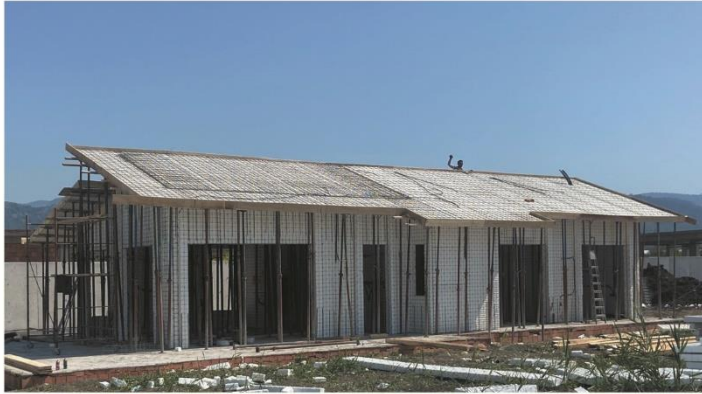
Both wall faces are being shotcreted with cement based mortar. Concrete is poured on the slab.
