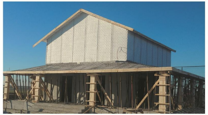
Zenon Panel Structures' static behaviour is monolithic, all walls transfer the load linearly to the ground.
