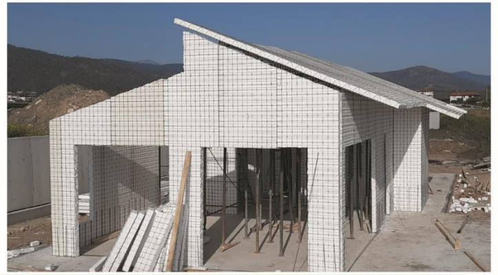
Panels are cut according to the project dimensions. All panels are connected to each other with meshes.
