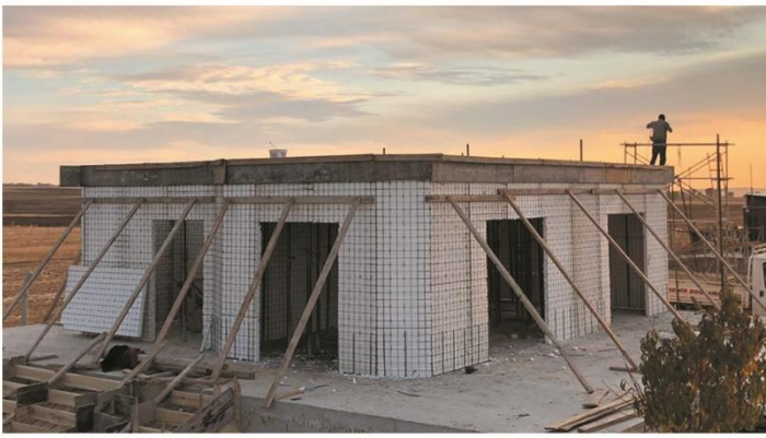
Zenon Panel Structures' static behaviour is monolithic, all walls transfer the load linearly to the ground.
