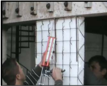
( a ) Shear Connectors
