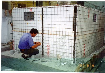
Photo 4. Specimen During Construction
